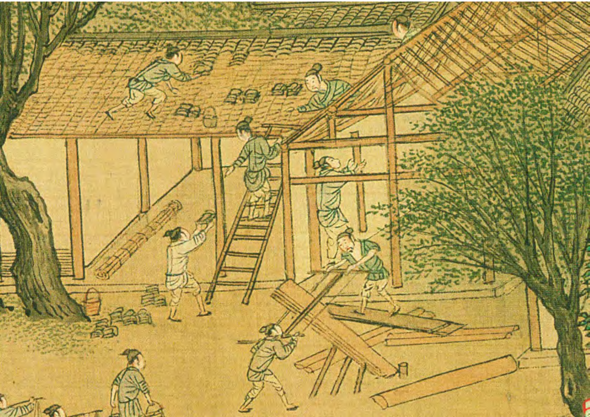
Plate7 Detail : house's building
