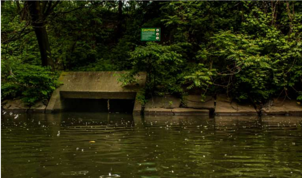
A CSO/Wet Weather Discharge Point on the West coast of the Bronx River near Tremont Avenue, New York. Photo: Adi Talwar
