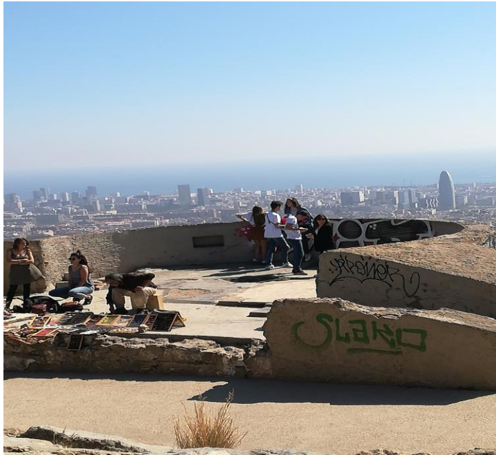
Remains of one of the anti-aircraft batteries of the Turó de la Rovira
