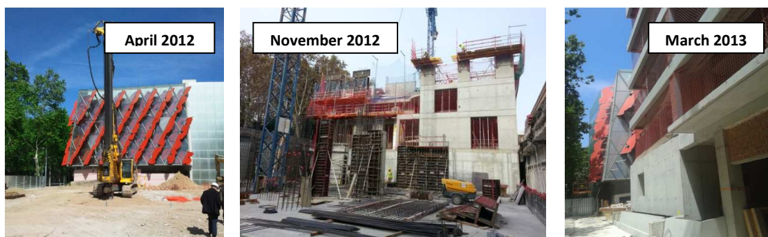
Figure I. Construction of the UPF Research Park (progress 2012-2013)
